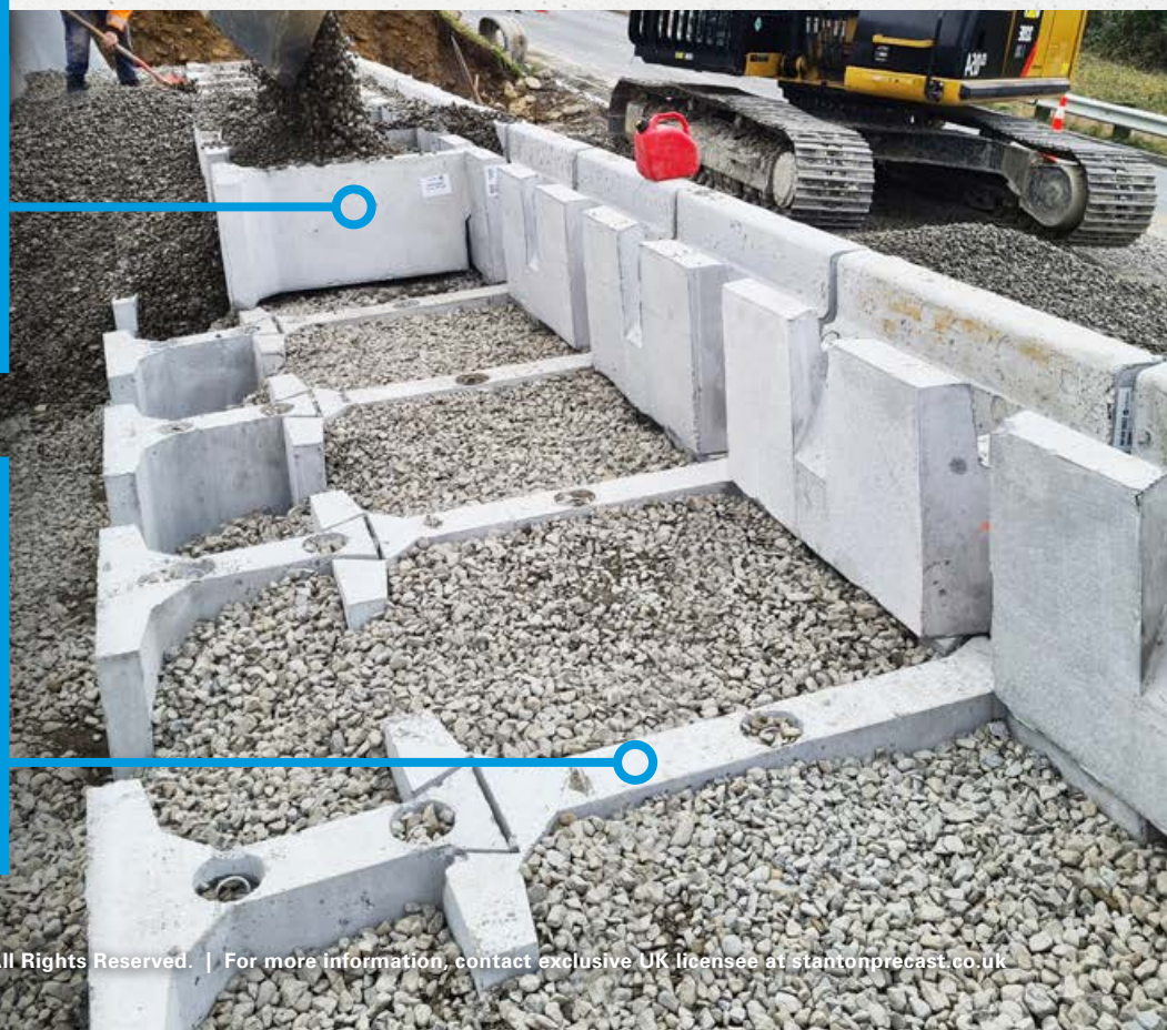
Gravity Wall with Extenders
